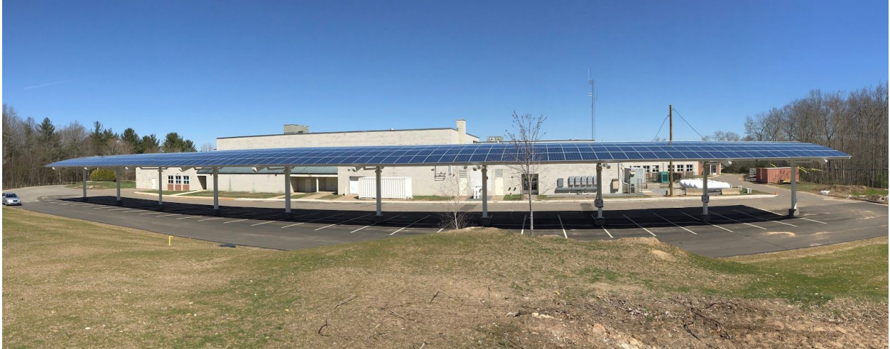
Carport Behind the Stafford Middle School
